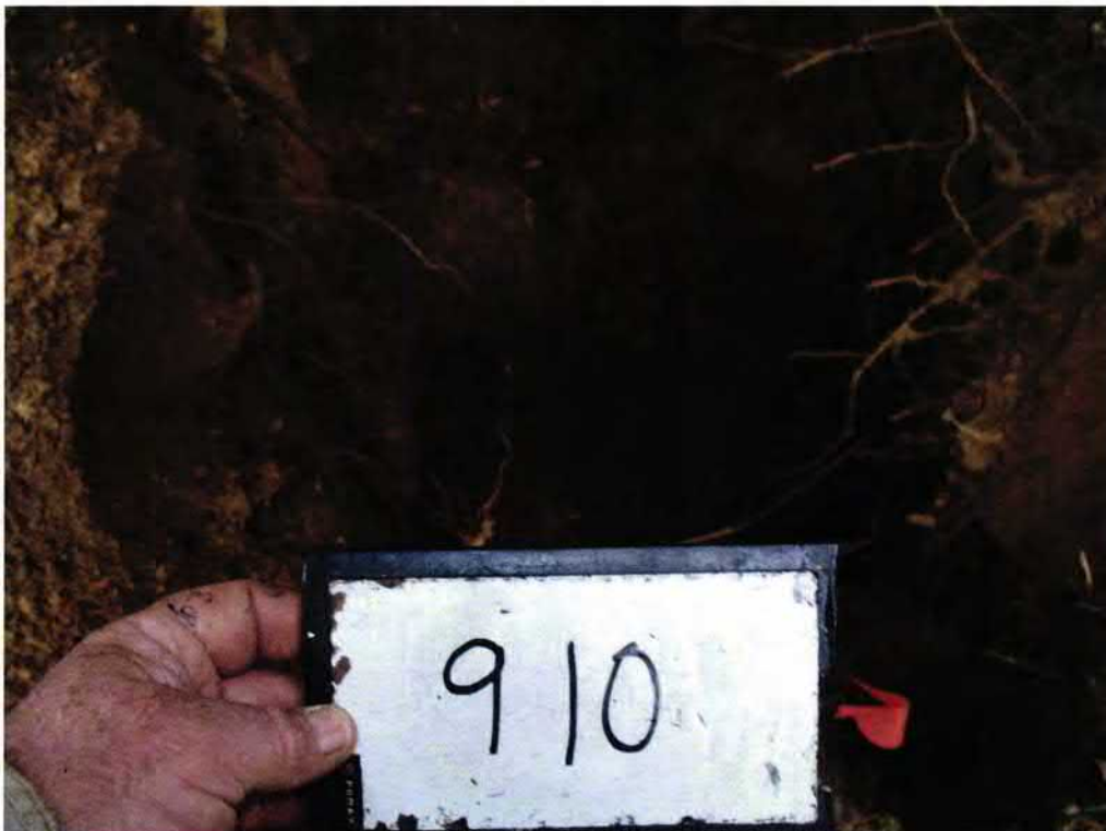
Picture 2: Tank pit after removal.
